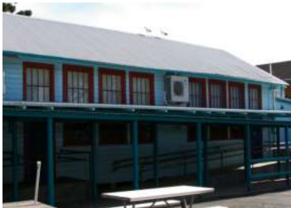
Figure 17: Typical arrangement of four double hung windows on the South-eastern facade of building B at Coffs Harbour Public School. ( Source: Conrad Gargett)
