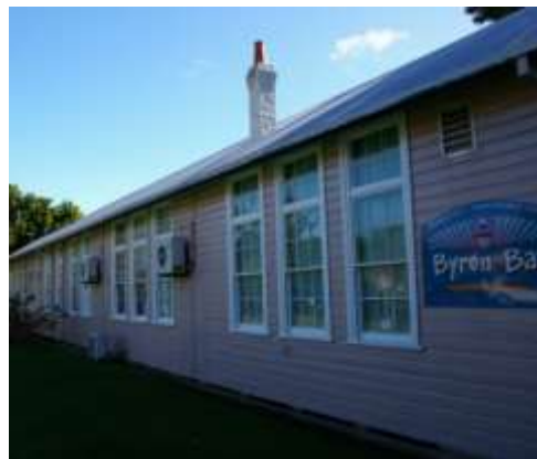
Figure 18: Typical arrangement of double hung windows on the south facade of building B at Byron Bay Public School. ( Source: Conrad Gargett)
